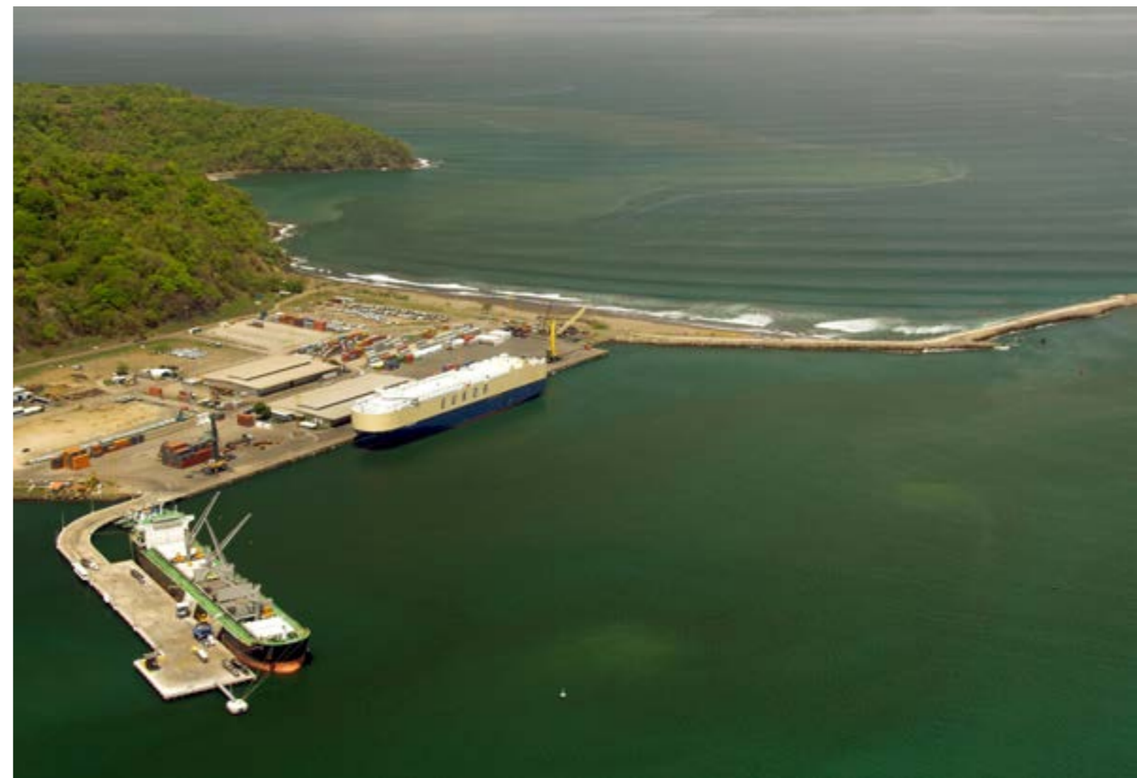
Caldera Port Terminal, Costa Rica.
