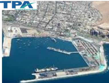
Terminal Puerto Arica S.A. (15% SAAM)
