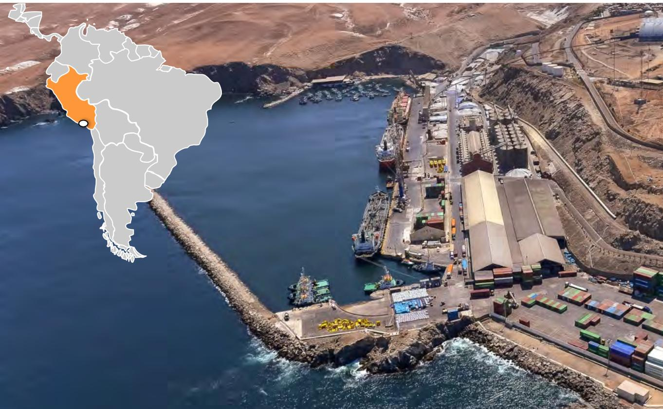
A terminal located in southern Peru, specializing in the mining industry from the central southern region. The terminal features a new dock (F) with transport capacity amounting to 1,500 metric tonnes per hour.
