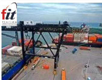
Florida International Terminal, USA
