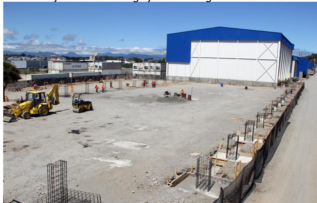
Construction of new cold storage facilities begins in Puerto Montt
